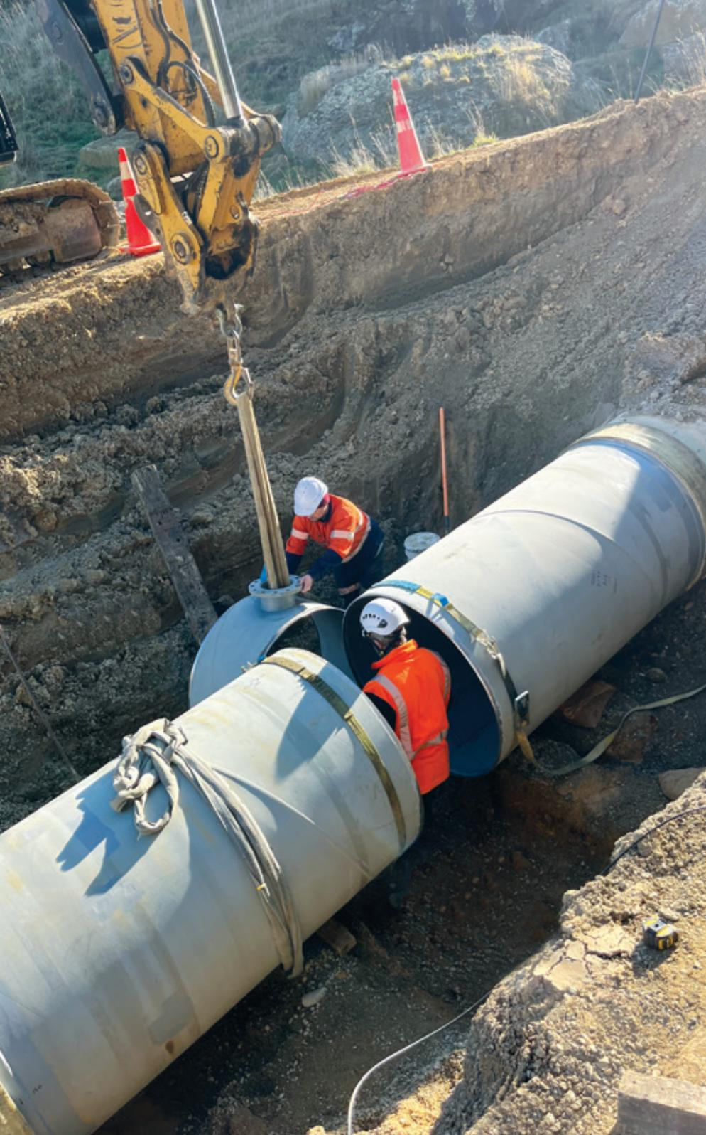
Pipe repair work undertaken by contractors at Queens Flat.
